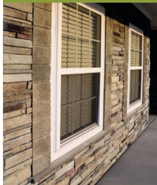
Wainscot cap as window sill
